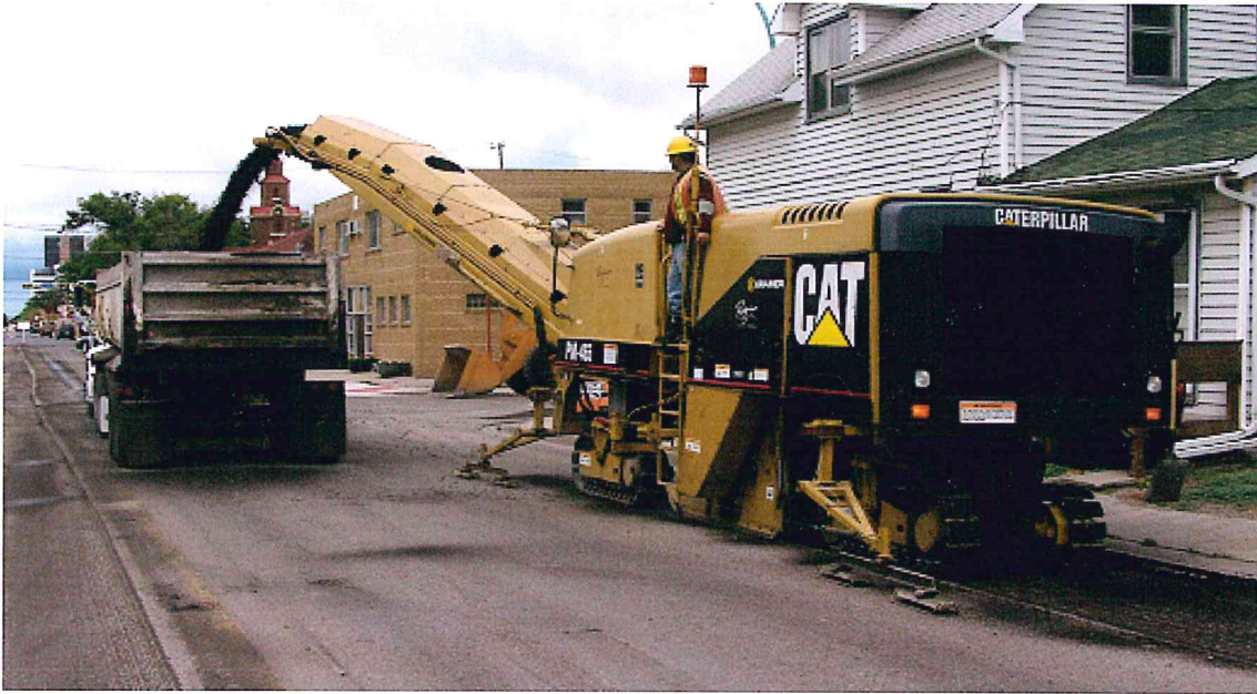
The asphalt paver crew performing precision asphalt cutting - preparing the road surface for repaving.
